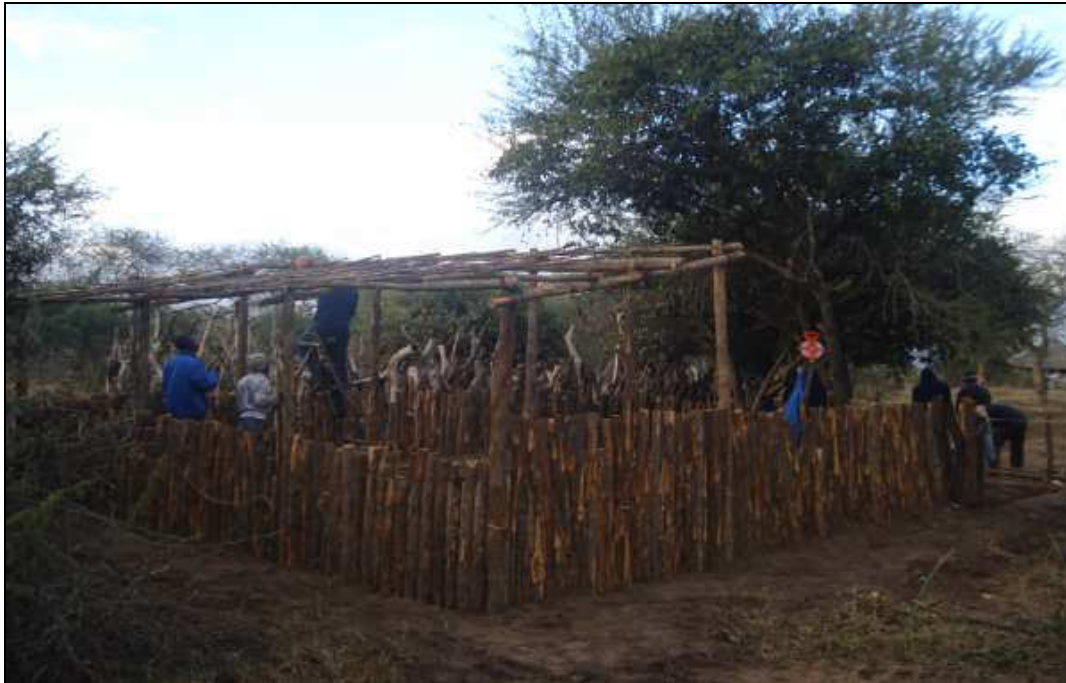
Picture 2: construction of improved goat keeping site in Chiuacaia community
